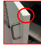
Damaged laminate cabinet
